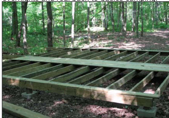
Tent platform construction in the Darrah Preserve
