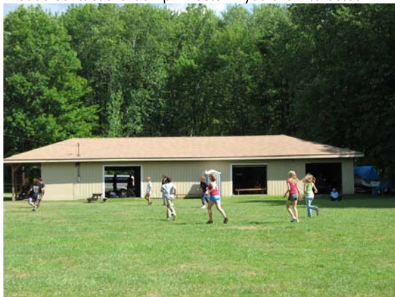
Say "good-bye" to the (green?) pole barn, it will soon transform too!
